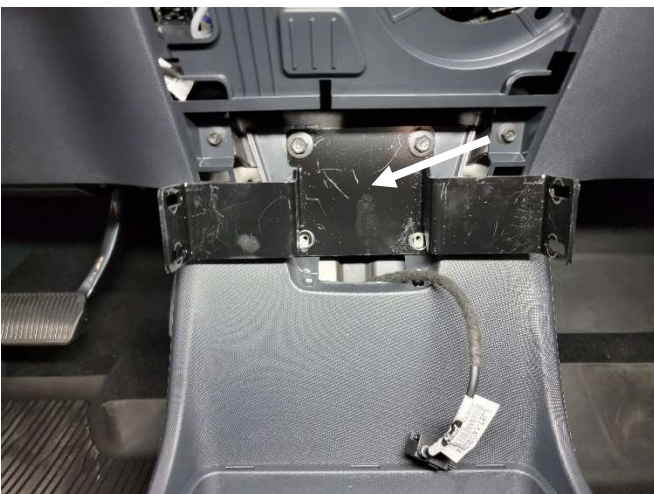
Attach the front mounting bracket using previously removed OEM fasteners.
