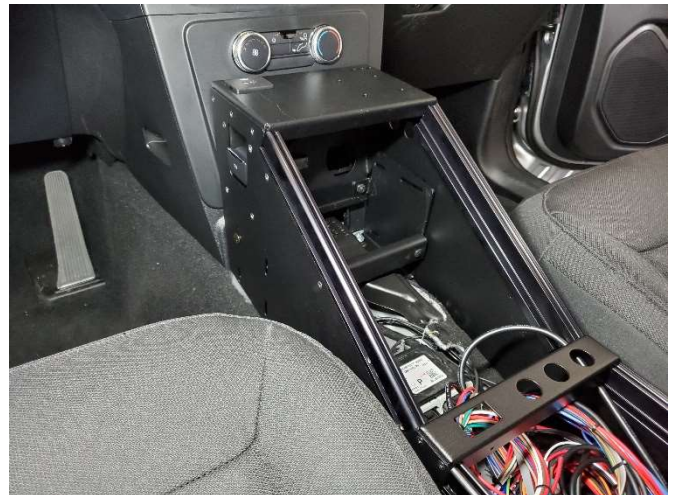
Relocate OEM USB module into top of console. Wire and install equipment as needed.
