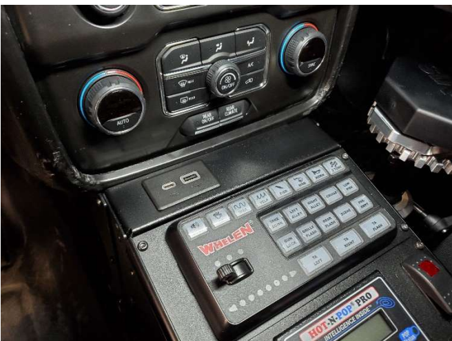
Install equipment into console.
