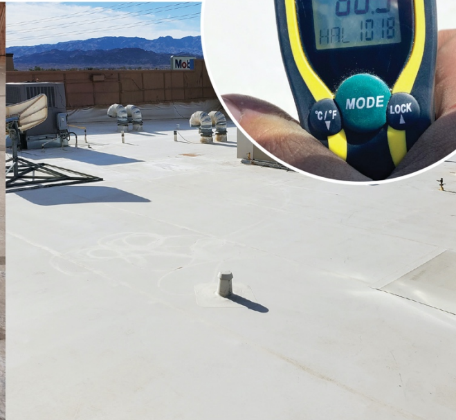
After coating air temp 99°F Surface temp 80.3°F
