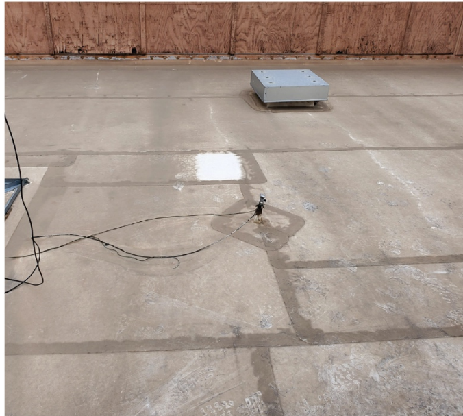
Before coating air temp 99°F Surface temp 154.6°F
