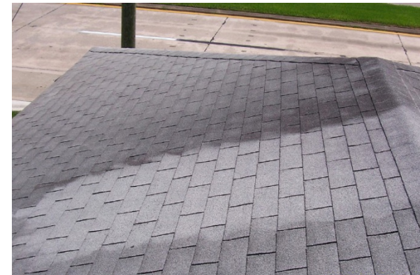
After 60 days area shows self cleaning in progress
