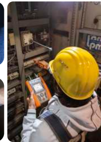
Start/stop measuring with remote lead PR400.
