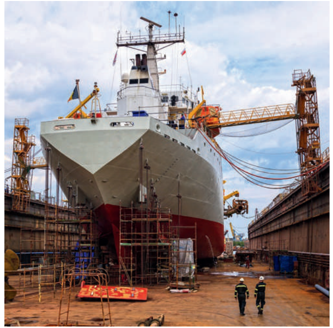
In floating voltage systems, e. g. with emergency power battery systems in marine engineering, the control voltage needs to be galvanically isolated from the battery voltage
