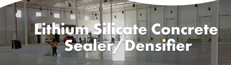
A premium lithium silicate sealer/densifier for concrete surfaces. LithSeal SC deeply penetrates and reacts with cured concrete. This reaction produces a calcium silicate hydrate within the concrete pores. Treated surfaces will remain breathable, reduce porosity, reduce dusting, reduce water permeability and increase abrasion resistance. When properly applied, LithSeal SC will not leave the whitish blush characteristic of other sodium silicate products.
