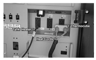
Figure C18 Heat Cord Connections
