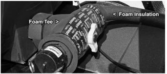
Figure C20 Foam Insulation
