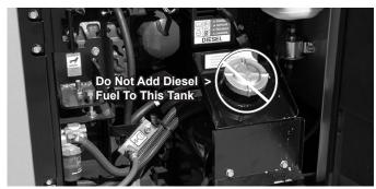
Figure C7 Generator Diesel Tank is Disconnected
