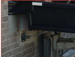
CHAINS/BRACKETS- Chains and brackets are provided on every dock-to-ground ramp. Once the brackets and chains are securely fastened to the face of the dock the ramp is ready for use.
