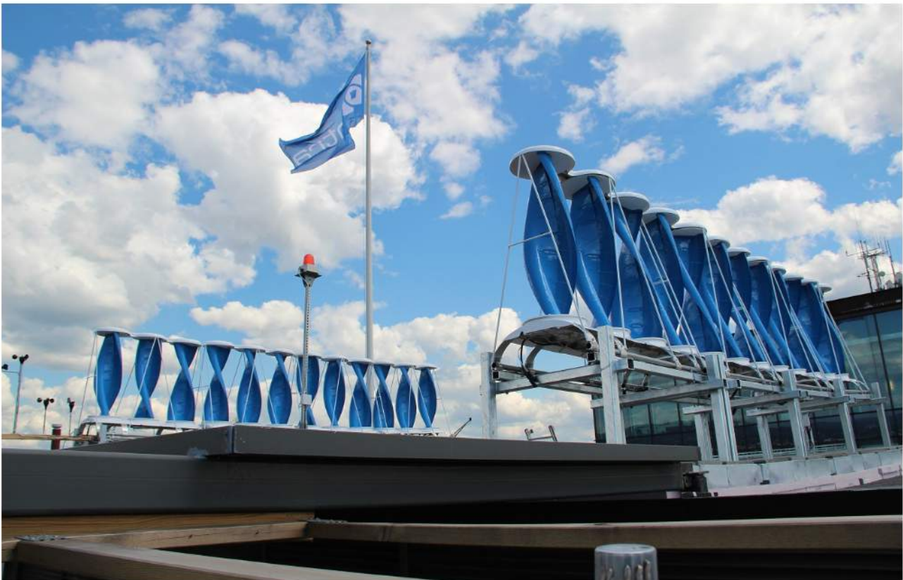
Figure 4: Installation of wind turbines and wind measurement devices (PHOTO: SINTEF Byggforsk)
