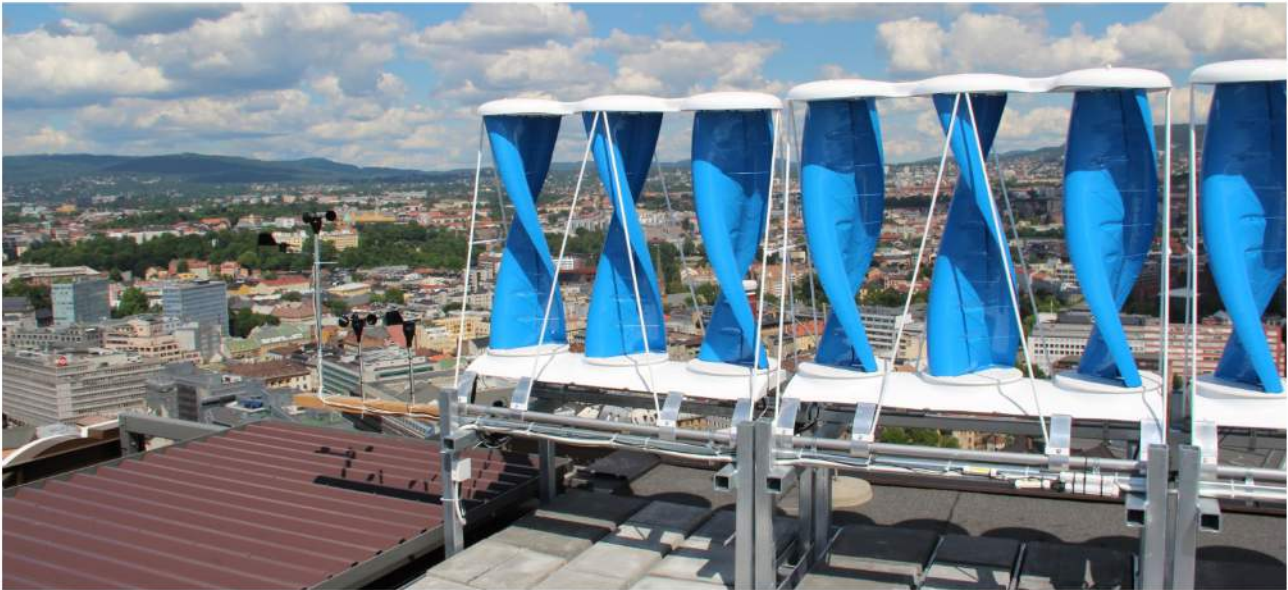
Figure 7: Wind measurement devices (PHOTO: SINTEF Byggforsk)
