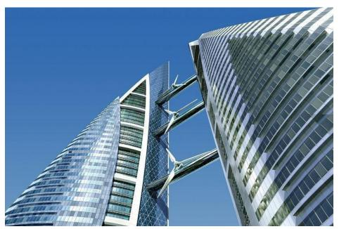
In keeping with its net zero design and construction concept, the ToB would also be outfitted with a series of vertical axis wind turbines (VAWT) and other wind scooping features that would enable the gigatower to function as a wind farm in its own right and one able to generate enough electrical power (160 GWh+) to replace the 26 Nordex N80 wind
