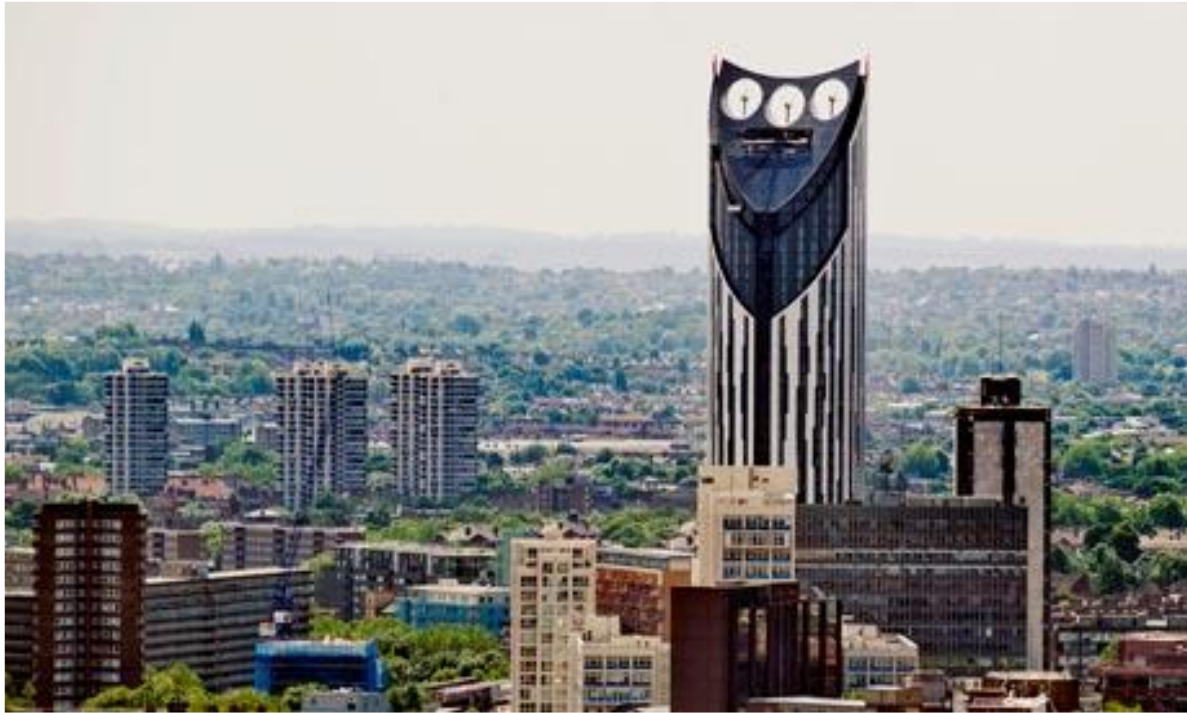
Figure 23 Strata Tower with 3 HAWT [112]
