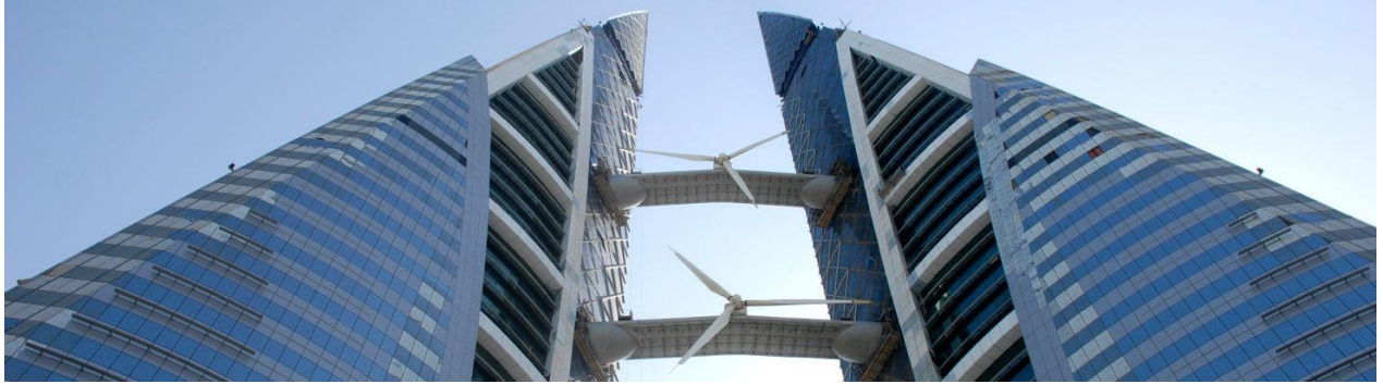
Figure 21 First large-scale building-integrated turbine project World Trade Centre in Bahrain, 2008. [110]
