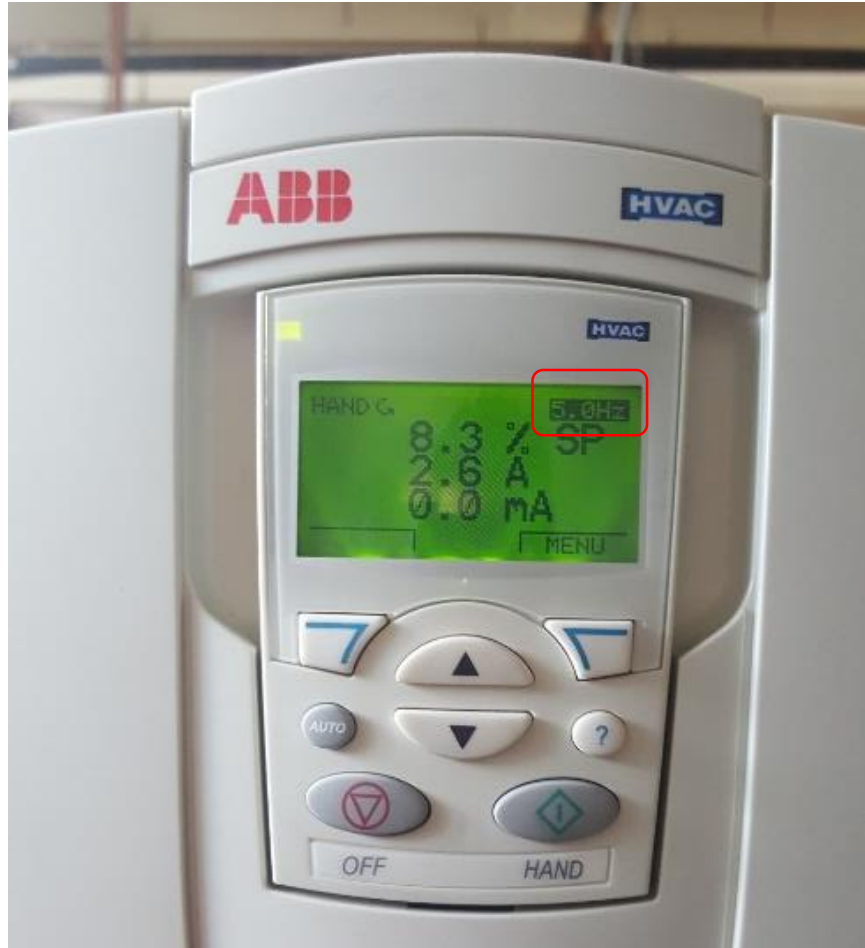
Figure 47 Fan speed set on 5.0 Hz. (Photo by author)
