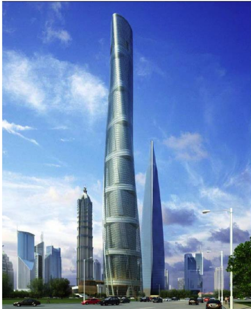
Figure 16 Shanghai Tower Site, Lu Jia Zui[107]
