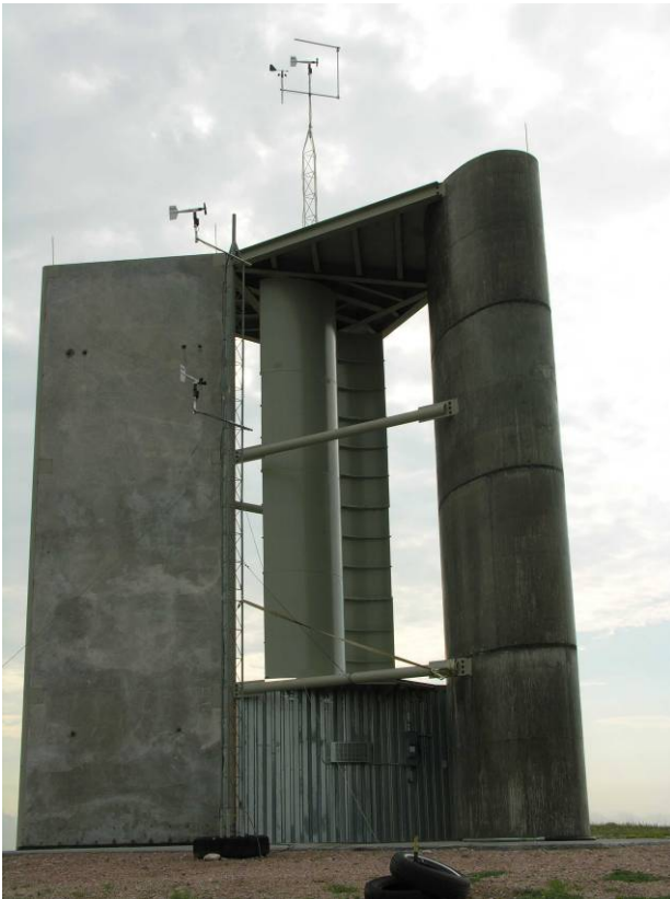
Figure 3: TMA Vertical Axis Ducted Savonius Wind Turbine
