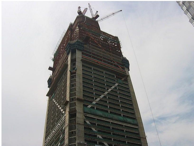
Figure 12. Shanghai World Financial Center during construction showing central core, corner megacolumns, perimeter diagonals, and belt trusses; diagonally arranged outriggers are hidden inside (photograph in public domain).
