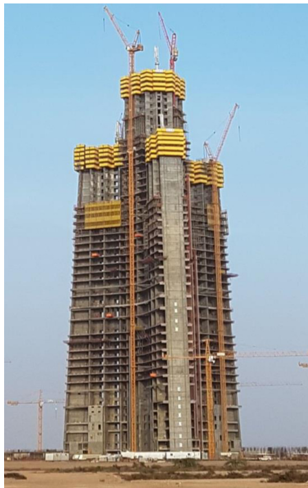
Figure 15. Jeddah Tower under construction (photograph in public domain) and its simplified structural plan showing central core, extended shear walls, thickened end flange walls, and fin walls.
