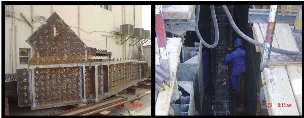
FIGURE 10 – PREFABRICATED BUILT-UP STRUCTURAL STEEL MEMBERS IN CENTER CORE WALL
