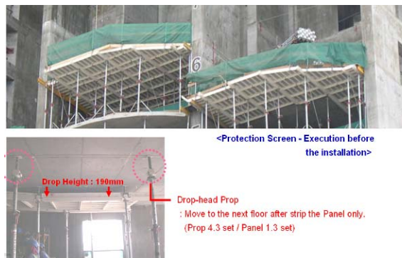
FIGURE 13 – TYPICAL SLAB FORMWORK SYSTEM
