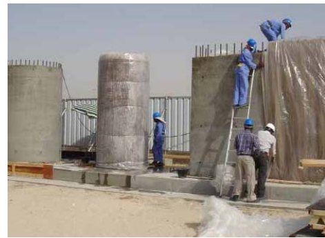
FIGURE 8 – HEAT OF HYDRATION MOCK UP TEST
