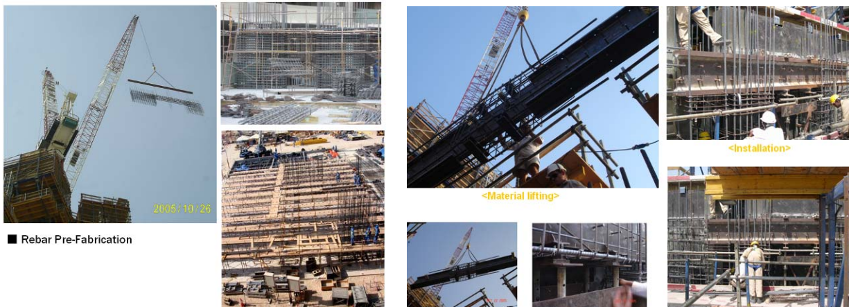
FIGURE 11 – REBAR PREFABRICATION FIGURE 12 – COMPOSITE LINK BEAM INSTALLATION
