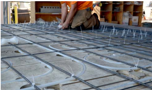
Figure 26 – PEX Tubing being Tied to Soffit Cage
