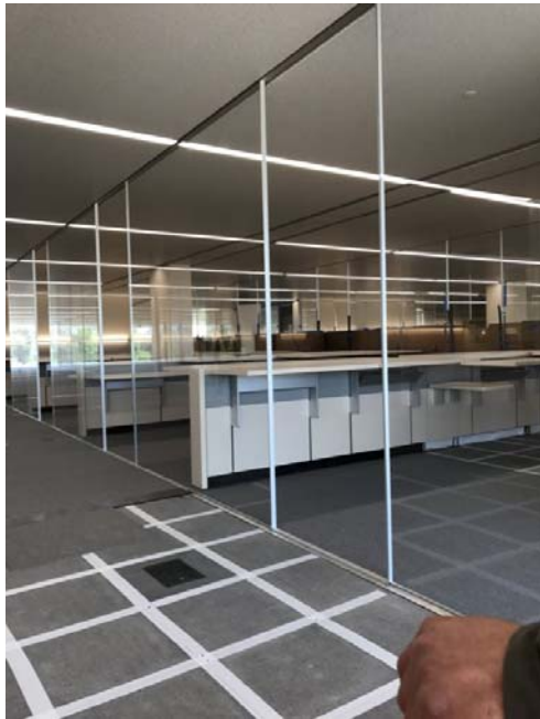
Figure 5 – Full Height Glass Partitions
