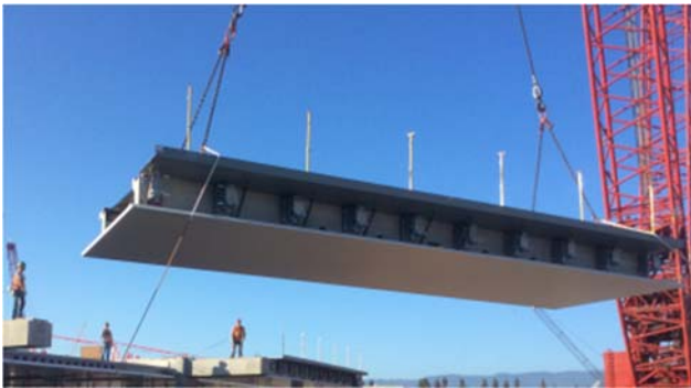
Figure 30 – Void Slab Hoisting with Pre-Installed Canopy Blade Brackets, Handrail, and Edge Form
