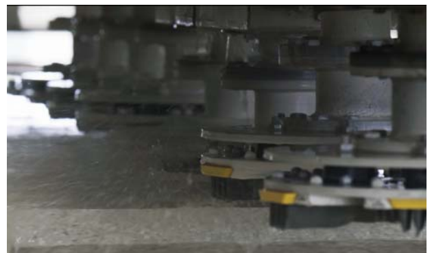
Figure 25– Honing of Void Slab
