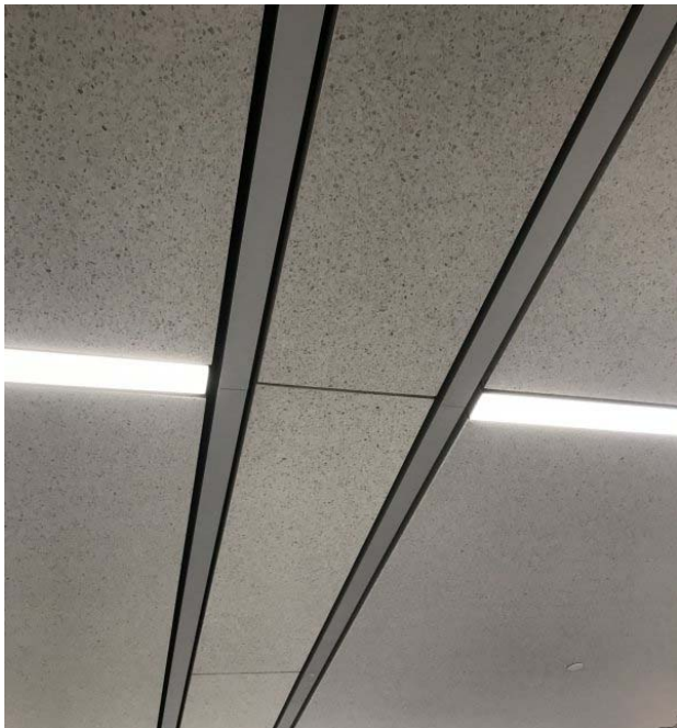
Figure 38 – Erected Void Slabs
