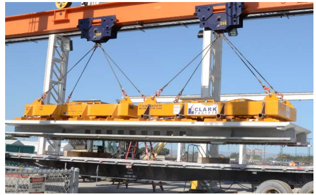
Figure 23– Vacuum Lift of Inverted Void Slab
