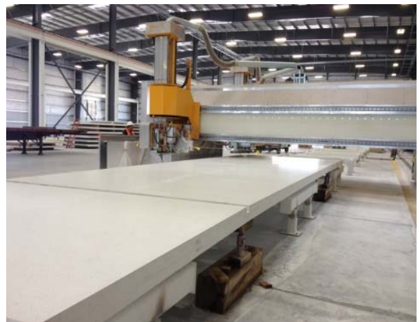
Figure 24– Honing of Void Slab
