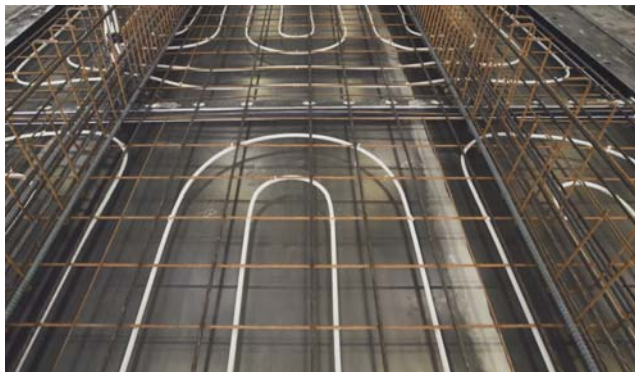
Figure 27 – PEX Tubing in Precast Form
