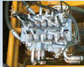
▲ Including new control valve, increased the diameter of hydraulic piping diameter
