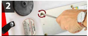
Remove screws from bottom of sign and remove the old lighting system.
