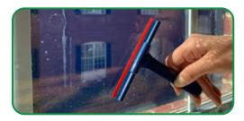
O2 Spray the film & window. Apply either side of the film to the window. Then spray again. Squeegeeing from center to edge, remove as much solution out from under the film as possible.
