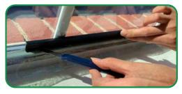
Using the cutting stick along with the knife. Carefully trim off any excess film.
