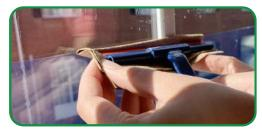
To finish, spray again then wrap the squeegee with napkin and begin squeegeeing from the center to the edge. Apply firm pressure to ensure sure all bubbles are removed from under the film and that all edges are flat.
