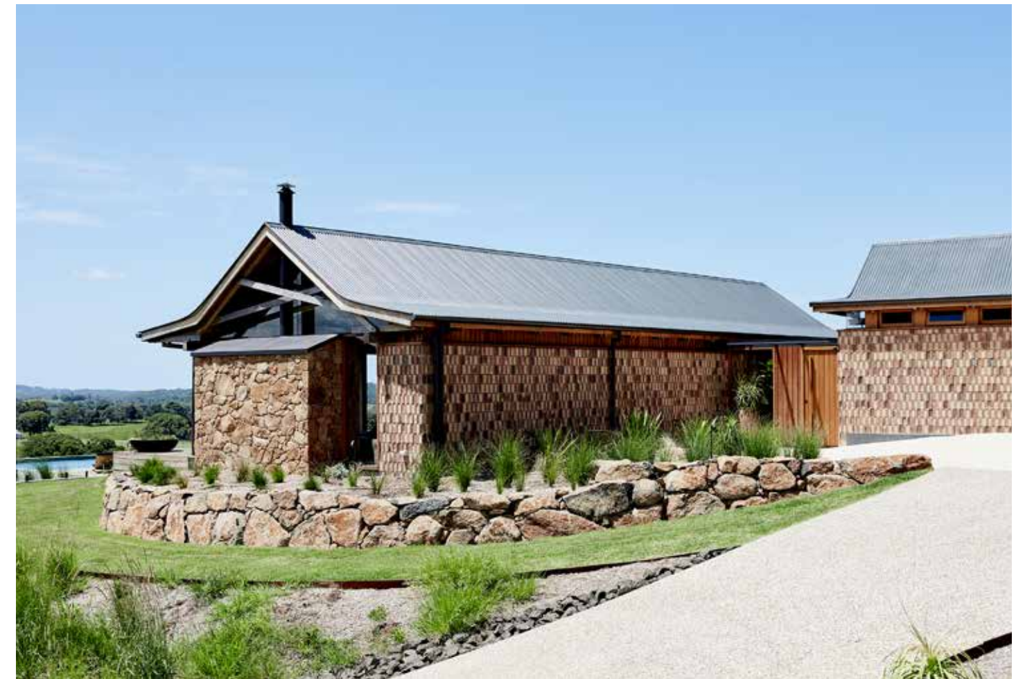
The off-grid design strengthens the connection between architecture and the landscape, eradicating its operational footprint without compromising on contemporary comfort.
