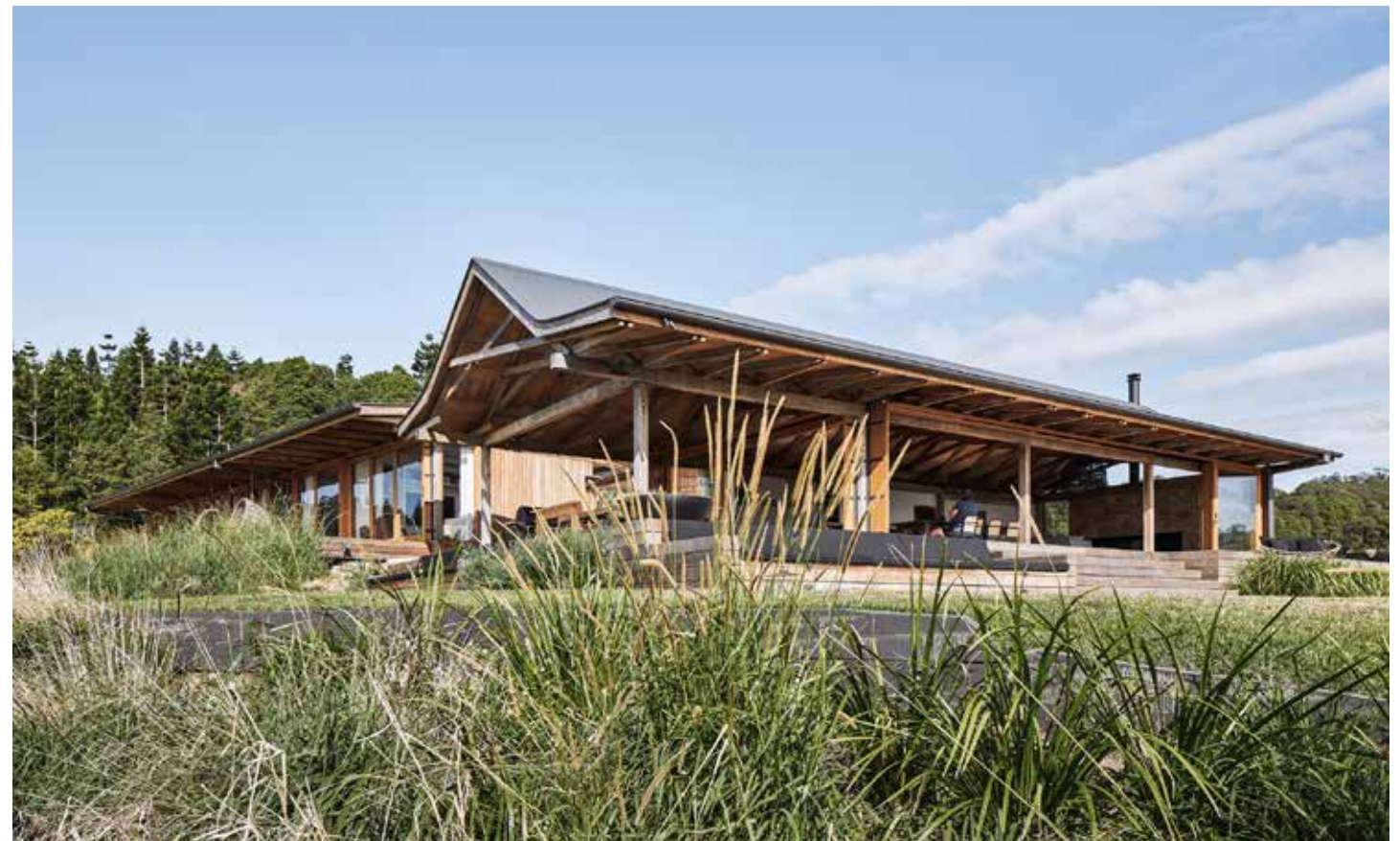
Set deep within the landscape, House for Walker Farm captures the essence of Myocum's distinctive rural identity. opposite Structure becomes the prominent form, with trusses reminiscent of traditional shearing sheds.
