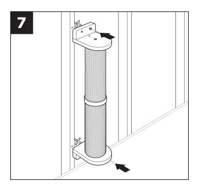
Insert toggle bolts into drywall. Pull the post away from the wall as you drill to ensure the toggles tighten.
