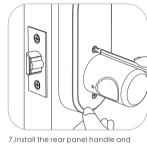
6. Insert the rear handle with the fittings into the toggle lever
