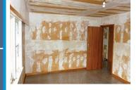
Apply one coat of pre-wallcovering sealer, following the manufacturer's instructions. Sealing the surface prevents over absorption of size and paste, staining and shadowing transferring through the wallcovering and plaster repairs becoming soft and falling off.
