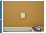
Apply one coat of pre-wallcovering sealer. Follow the manufacturer's instructions. This will prevent colours showing through after the wallcovering has been applied. Sealing the surface prevents over absorption of size and paste and prevents the acrylic paint from softening and the new wallcovering falling off.
