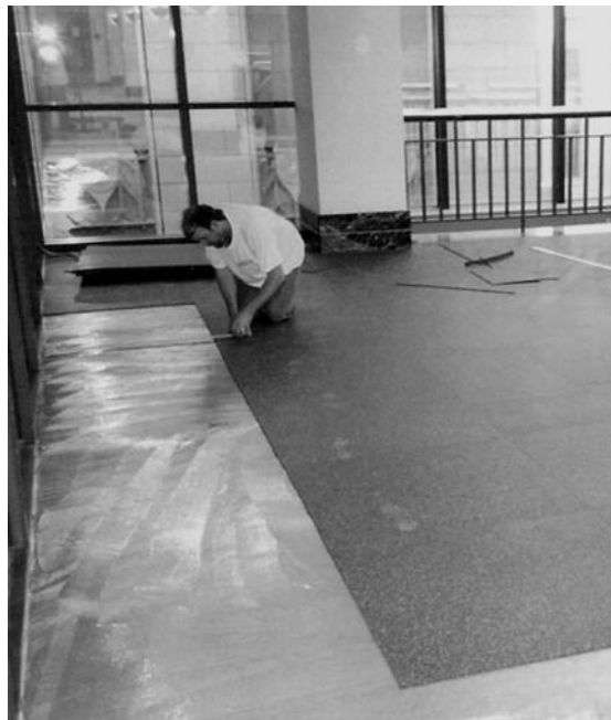
Square Cut / Glue Down Installation
