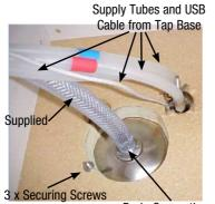
Drain Connection at Font, install supplied clamp here
