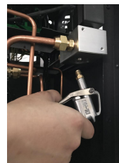
Cleaning before installation
