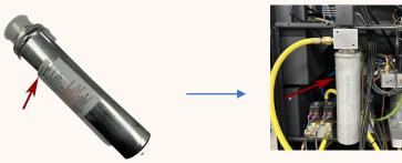
• Note down the code on the new filter, you'll need it when resetting the machine later
