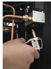
Cleaning before installation
