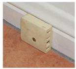
This is one of the most common technology on old residential or commercial areas. The optic fibre is delivered to a distribution point in the street and then is delivered with copper to the first socket of the premises.
