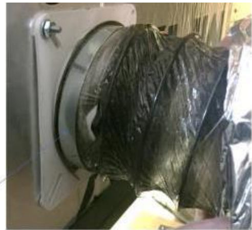
Connect the 4" insulated ducting inside liner to the heater intake and exhaust using screw clamps as shown above
