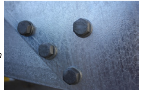
Lockinex branded structural connection bolts. Torque to 225 N/m
