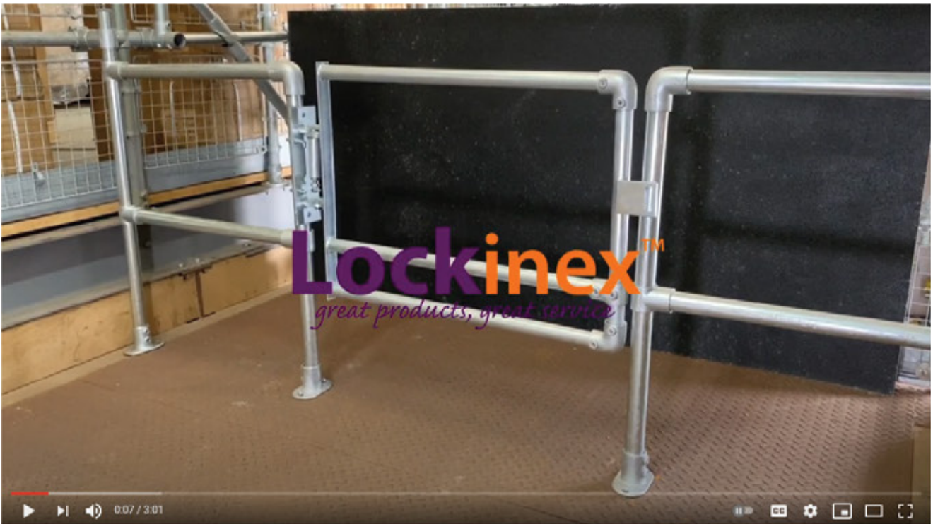
How to Install a self closing safety gate - Lockinex UK
