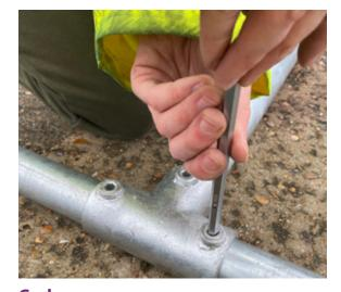
**Grub screw**Quick tightening/fastenings.
