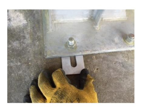
Trouser Shim being inserted under a base plate to align and level the vertical post.
