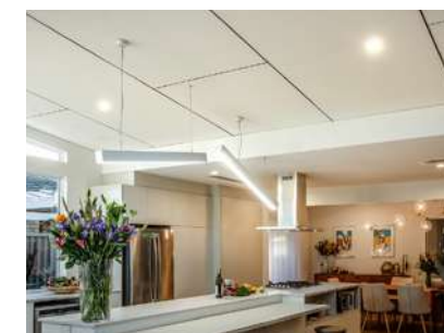
Versilux™ Lining Ceiling or soffit lining with black express joint accessory.
