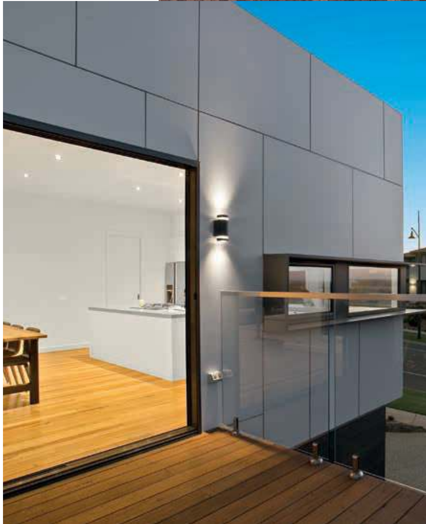
Pivot Homes Silvertop Ash decking
