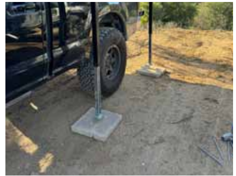
PLACE CONCRETE PAVERS UNDERNEATH THE LEGS
