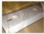
Place the cover on top of the tee bar grid.
