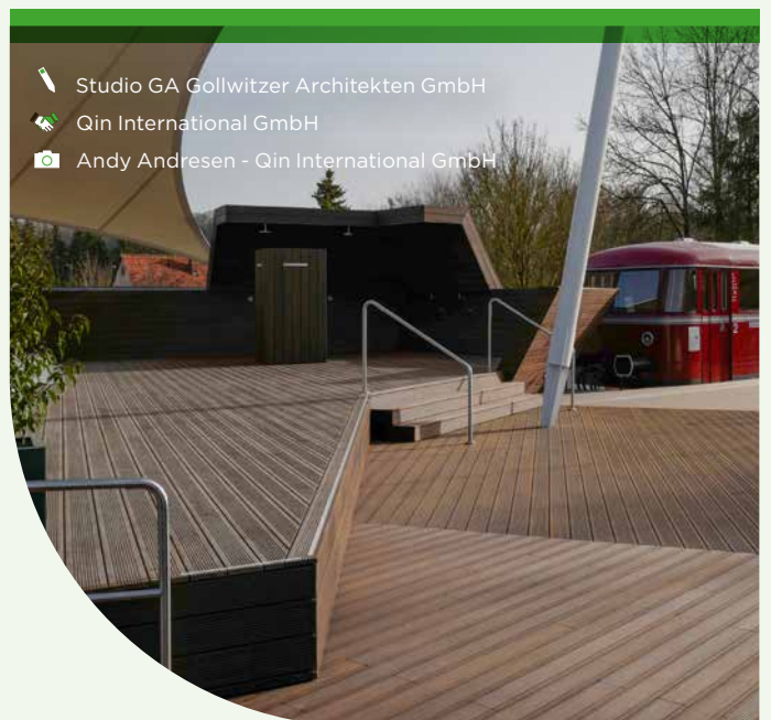
Altmühltherme Wellness decking with FSC® certification installed on a steel structure - (1000 m 2 ) Treuchtlingen, Germany
