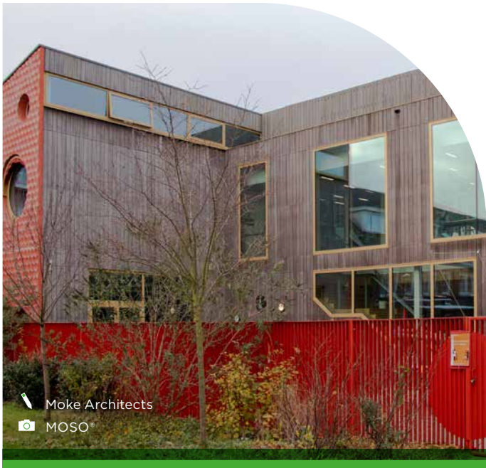
Public Elementary School "IKC" photo taken 5 years after installation - (320 m 2 ) Amsterdam, The Netherlands
