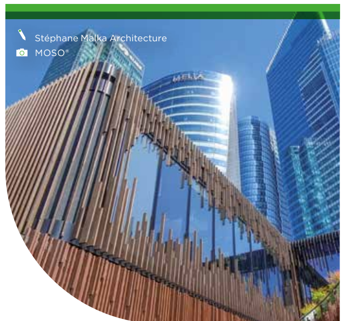
Oxygen La Défense Photo taken 4 years after installation (5500 m) Paris, France
