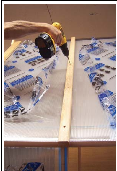
installing wood caps
