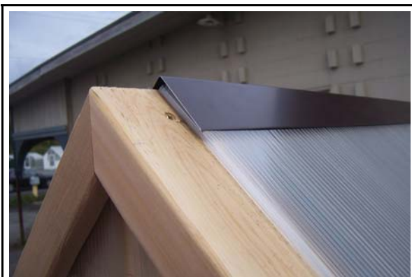
metal flashing along ridge
