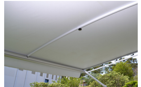
The curved design prevents water pooling.
