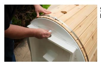
Screw the short pipe into the drain hole on the bottom of the tub.
