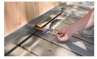
Using a pipe wrench or adjustable wrench, tighten the garden hose connector (if ordered) onto the valve.
