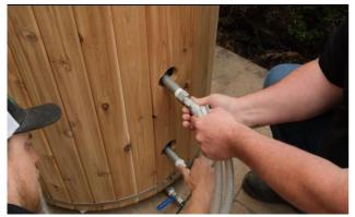
Connect the other ends of the chiller hoses to the tub. The hose from the outlet of the chiller will connect to the higher pipe of the tub and the hose from the inlet will connect to the lower pipe.
