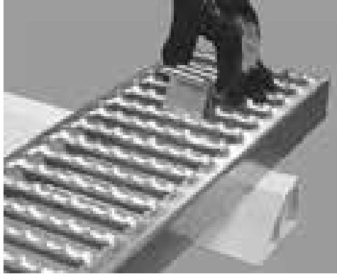
Position the grating on the Unipier sleeper support and insert the appropriate size hold down clip (G639, G607, or G620).
