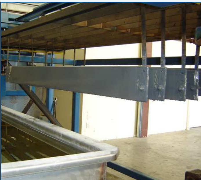
Epoxy Coating System
