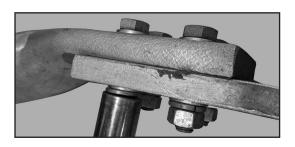
Step #11 Coat the dead-end terminal pad with conductive electrical joint compound.
