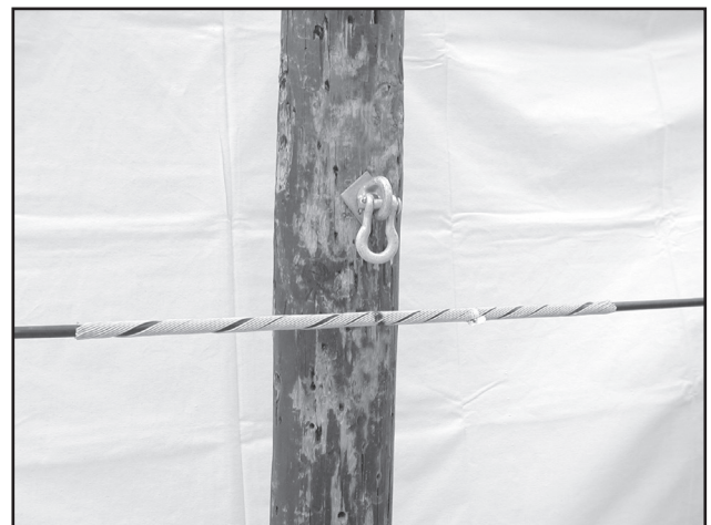
FIGURE 15 - STRUCTURAL REINFORCING RODS INSTALLED
