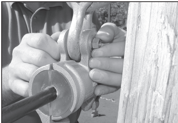
FIGURE 10: INSTALL LOCK NUT
