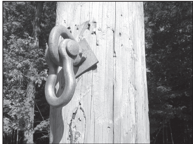
FIGURE 4 - EYE NUT 5/8" & ANCHOR SHACKLE OPTION
