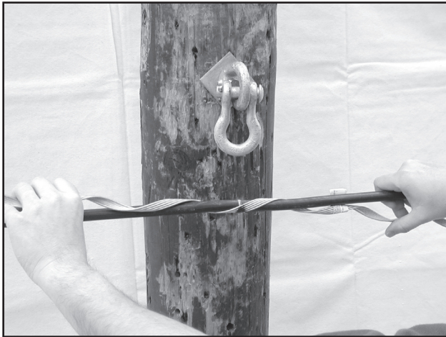
FIGURE 13 - ALIGN FIRST SUBSET
