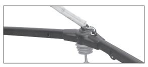
Step #2 Apply pressure to the top of the RPC using the hot stick and completely snap it over the conductor. Another stick can be used to snap the legs into place.
