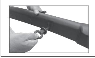
Step #4 Completed installation of the RPC for conductor angle with a tie top insulator.
