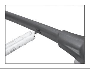
Step #4 Completed installation of the RAPTOR PROTECTOR for the conductor angle with a tie top insulator using hot sticks.
