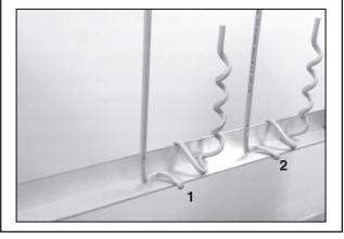
Step #5 Slide the second deterrent to position it next to the first, placing the helical upright behind the straight upright of the first unit.
