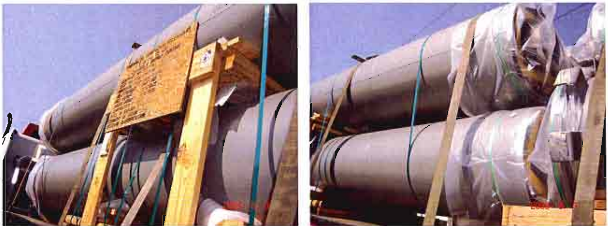
Relocating Bus Duct from storage to job site
