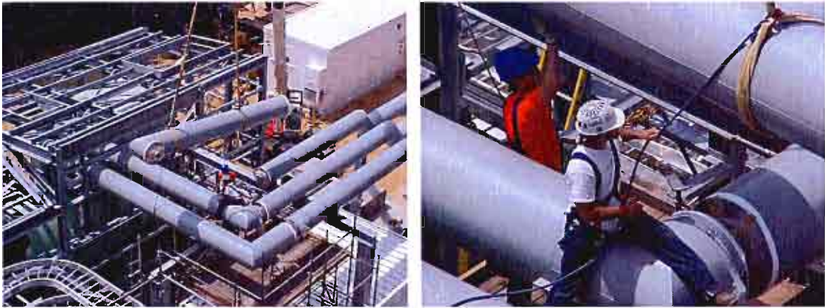
Preferred method of lifting and guiding bus duct into place
